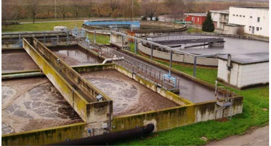
The Formellino plant purifies 1000 m<sup>3</sup>/hour of water diverting it from water flowing to the Lamone river.
